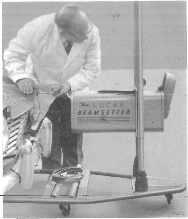
Fig. 49. Using Lucas beamsetters
